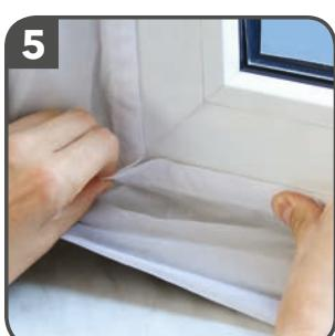
Stick the narrow **side B** (zipper is closed) from the middle to the left and right side or to the up and down side to the casement.
